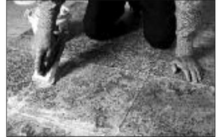
Apply the acrylic grout in to the tile joints with the narrow edge of the rigid rubber float. Firmly pack each tile joint so as to leave no voids or skips. As each tile joint is grouted, remove excess grout from tile edges with the stiff edge of the float pulled in a 45° angle across each joint. Grout only in small increments and clean each section as you go. Never apply grout in an area greater than 20 square feet without stopping to clean.
