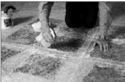
Use a dampened nylon scrubbing pad to loosen remaining grout from the tile surface. Wipe alongside the joint with the nylon pad to avoid removing grout from the joint. Do not use excessive water during cleanup.
