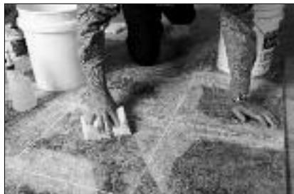
Use the special square edge sponge to remove the excess water and grout haze. Be certain to wipe diagonally across tile joints to avoid dragging grout from the joint. Rinse the sponge frequently and change the cleanup water frequently. Thoroughly remove all residual grout and grout haze before leaving the job. Dried grout haze is difficult to remove.
