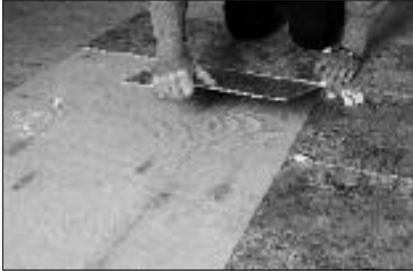
The desired grout width must be determined before tile layout begins. It's critical to include grout width measurement to tile size to ensure a balanced layout. Grout width should be at least 1/16" wide and no more than 1/4" wide. Commercially available hard plastic ceramic tile spacers may be used to maintain equal grout joint width.
