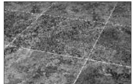
If a slight grout haze is noticed after 24 hours, it can be removed by scrubbing with the nylon pad and a solution of 1/4 cup ammonia in a gallon of clean water. Thoroughly rinse the area with clean water. **Do not use chemical grout cleaners.**
